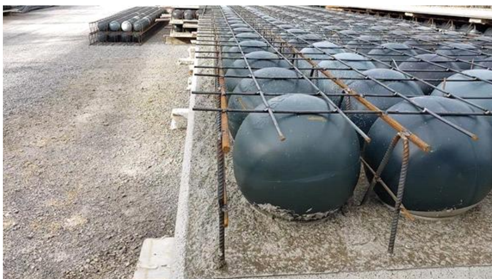
Figura 96 - Laje Bubbledeck.
